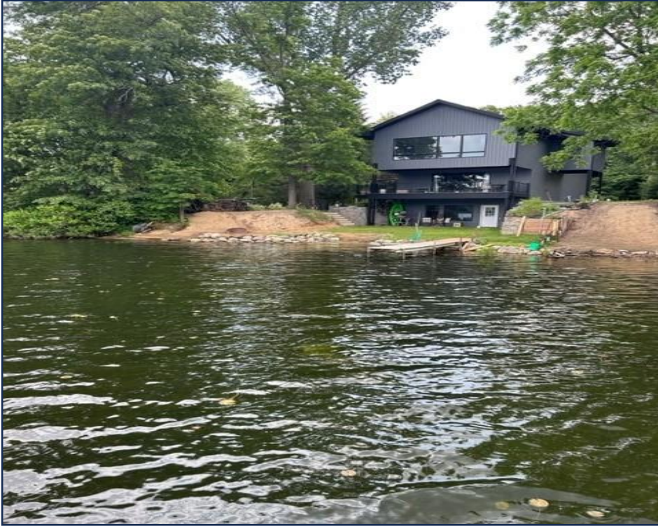
Figure 2. Erosion on a Perch Lakefront property (NOTE: This photo is for demonstrative purposes and is not meant to implicate any fault).
